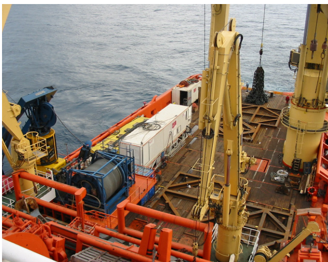
Modular AHC 175 / 40 / 6200 installed on deck of the SBM "Normand Progress"
